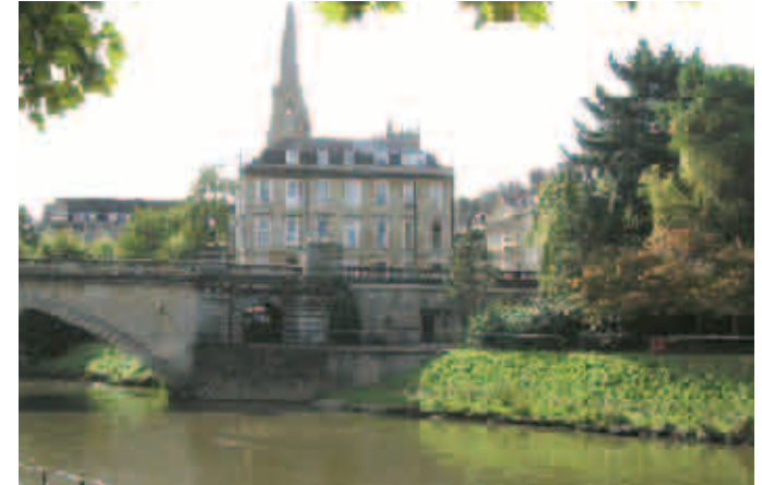
R3 North Parade Bridge looking back towards North Parade
