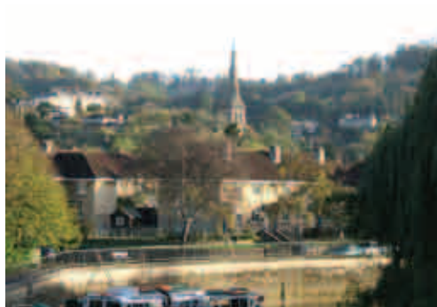
North Parade Bridge towards Bathwick and Prior Park
