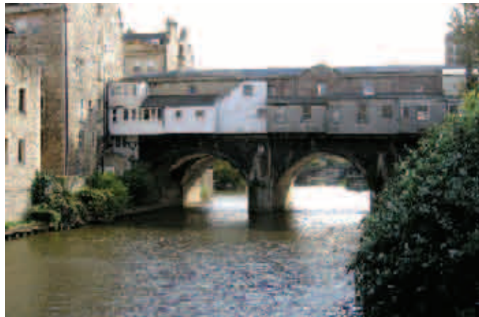
R5 Looking towards the back elevation of Pulteney Bridge.
